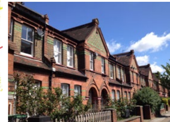
Low rise terrace, Noel Park Estate
