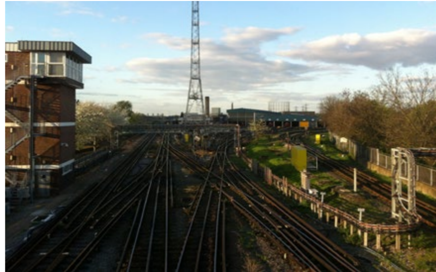
London Underground Victoria Line Depot, east of Northumberland Park Station
