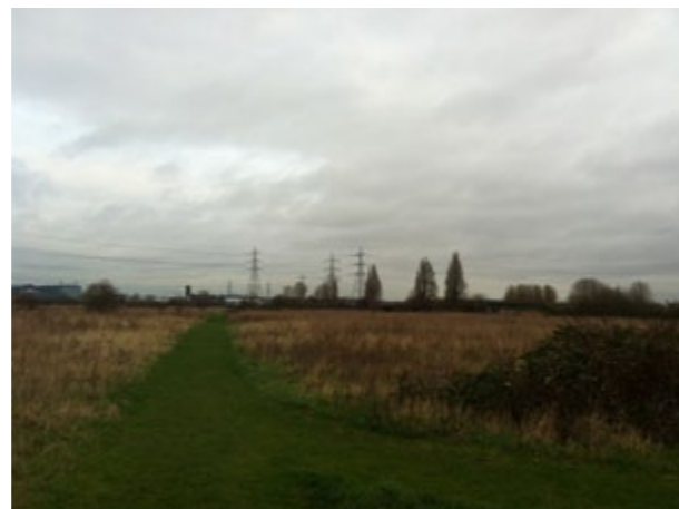
Lea Valley pylons 6 & 7
