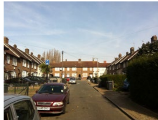
Regularly laid out houses in closes and squares in the west
