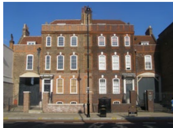
Grade II listed nos. 808-810 High Road, grand part of Queen Ann houses
