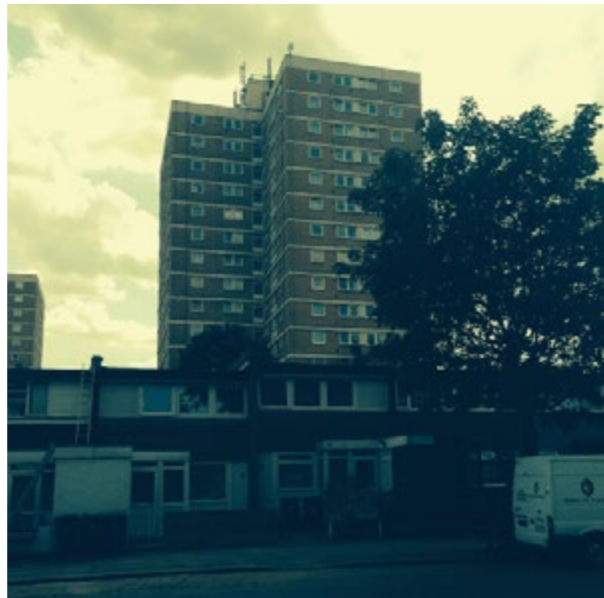
Slab and tower block estates comprising a mix of low and high rise buildings arranged pavilion style around open space connected by footpaths and access roads.
