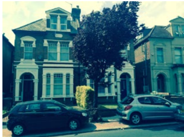
Grand villas and townhouses, tightly arranged, occupying medium size plots with strong vertical proportions, often with basements and raised ground floors.
