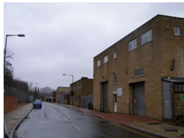
View along Western Road with some robust, solid brick industrial/workspace buildings
