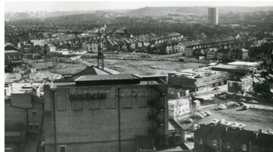
Aerial of Wood Green Shopping City under construction c1976
