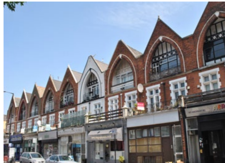
Arched retail terraces, Archway Road (East) at the southern end
