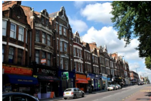
Mid rise retail terraces along northern end of Archway Road (West)
