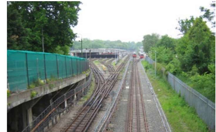
Railway Depot, northern end of Archway Road
