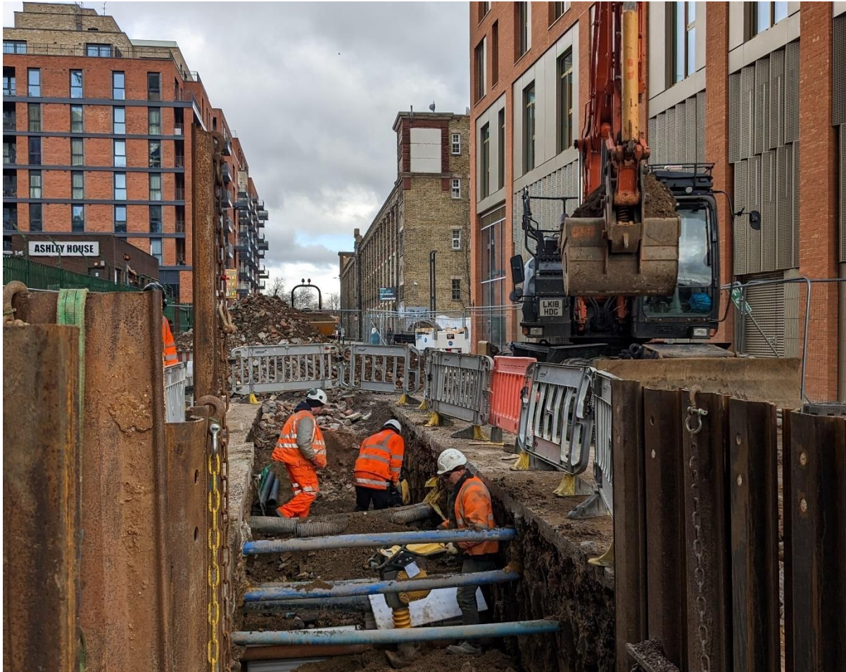
Figure 15: Installation of DEN pipework system in Ashley Road, Tottenham Hale.
