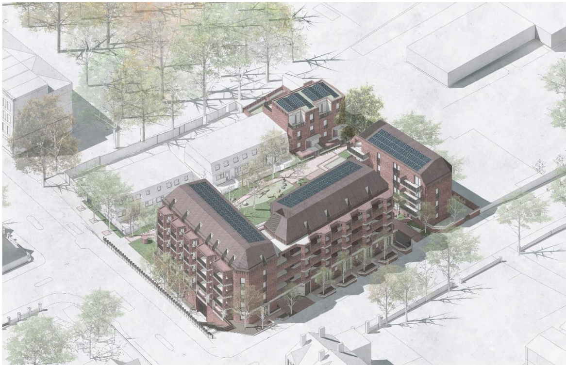
Figure 8: Cranwood House Scheme which includes erection of three buildings providing 41 homes which has been designed to Passivhaus standards, with very high fabric efficiencies and air tightness, triple glazed windows, a communal air source heat pump system, and solar photovoltaic panels on the roofs.
