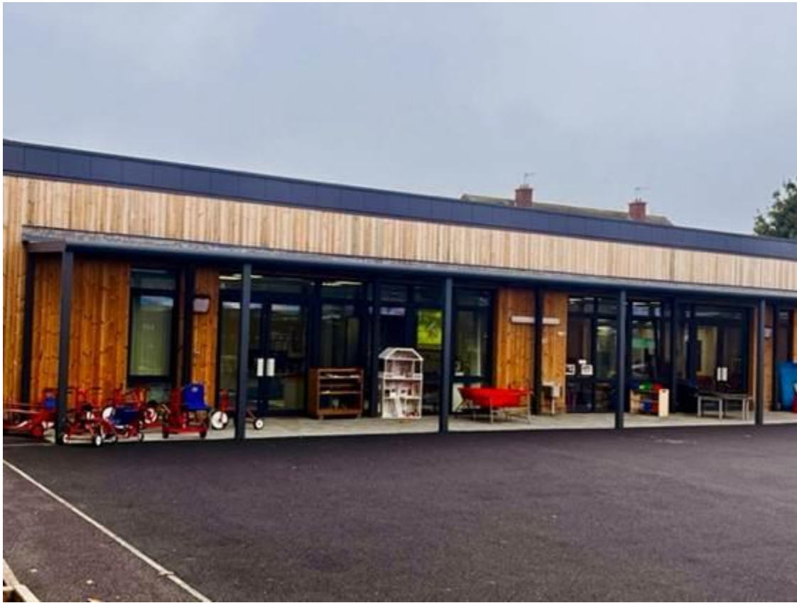
Figure 9: The new nursery building at Lordship Lane Primary School has two classrooms and is equipped with an air-source heat pump and photovoltaic panels which is a zero-carbon scheme.
