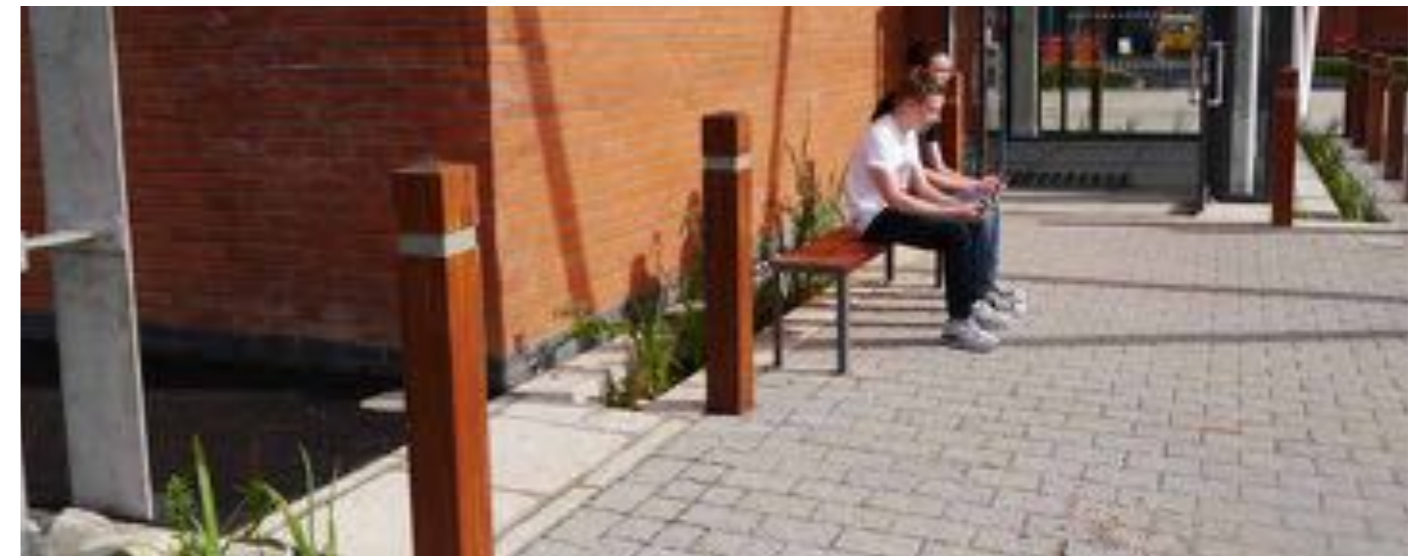
Permeable paving and planted open channels collect runoff from hard surfaces at Bewdley School, Worcestershire.
