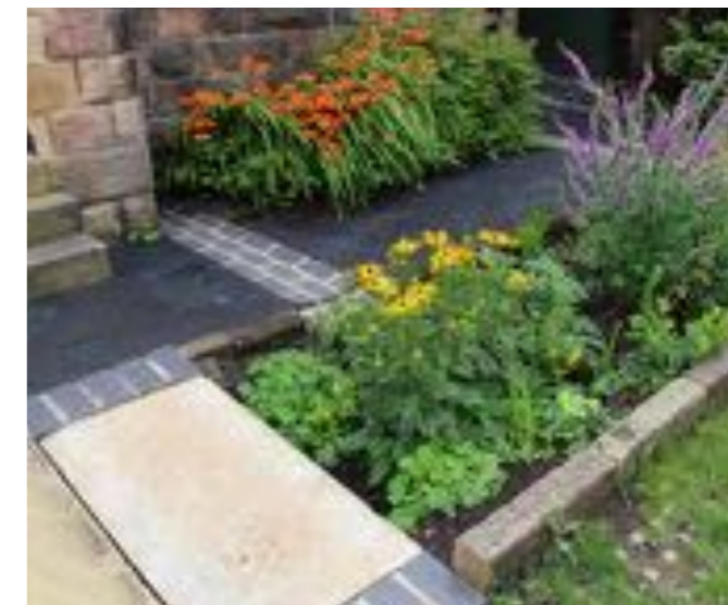
Strutts Centre, Belper. Brick channels collect roofwater for linear raingarden with garden style planting.
