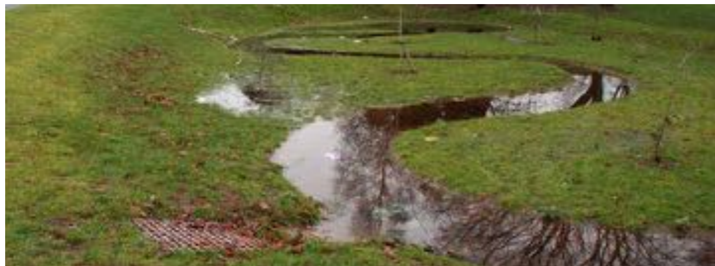
Controlled flows are released from one sub-catchment feature to the next, as here at Birchen Coppice Primary School, Kidderminster.
