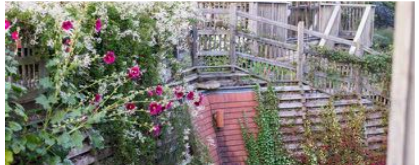
Springhill Cohousing, Stroud. Tile hung cascade conveys water through terracotta T-piece to lower level.
