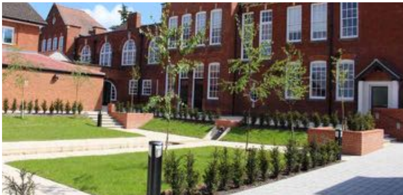
A sunken SuDS courtyard with solar water feature into a formal rill at Bromsgrove Civic Centre.
