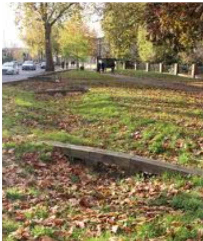
Rectory Gardens Rainpark, Hornsey. Forebays, swales and underdrained basins use SuDS turf (100-150mm) to filter runoff, with amenity grass for public use.
