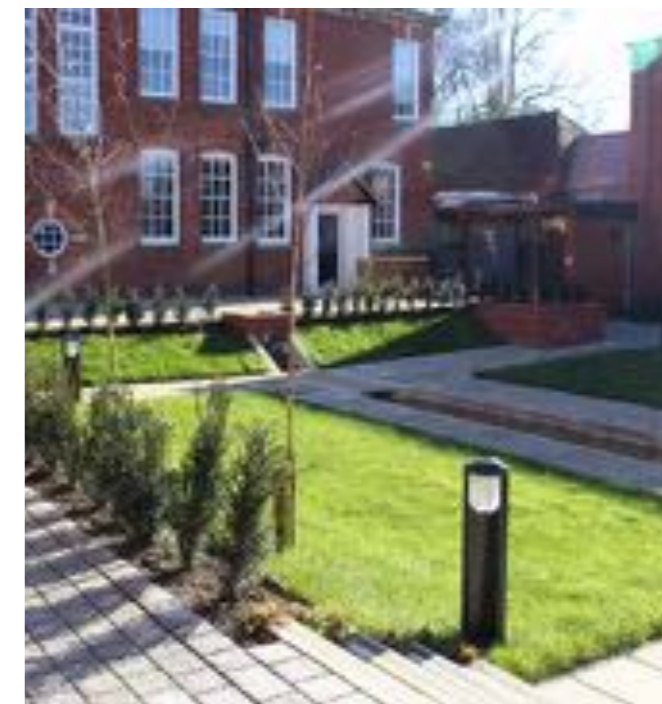
Parkside, Bromsgrove. Amenity grass shallow detention basin feature, integrated into site design, manages occasional extreme rainfall.
