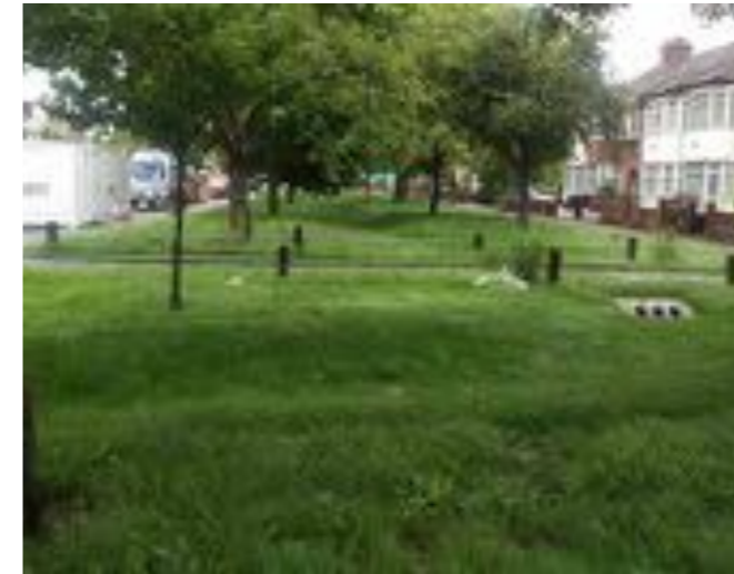
Highway runoff is intercepted using a chute gully and taken into a conveyance swale at this retrofit SuDS project. Devonshire Hill, Haringey.
