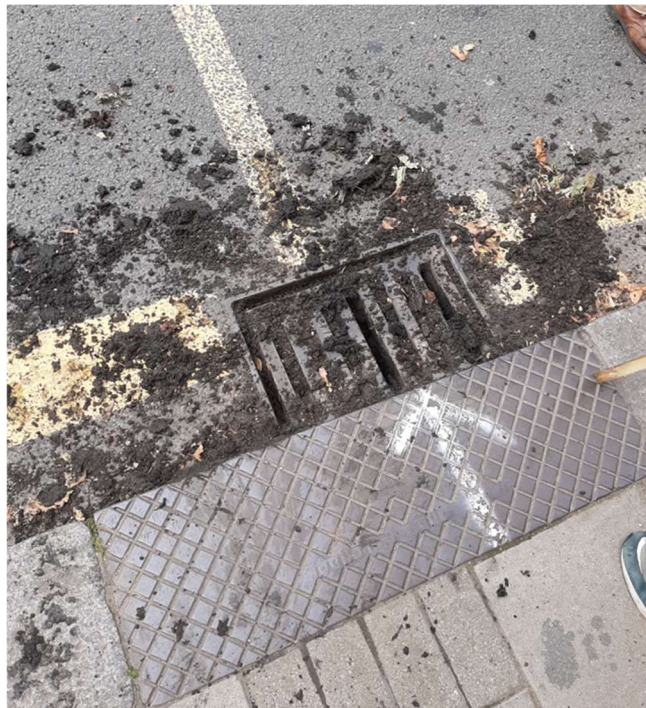
Figure 5-6 Failed attempt to unblock gully outside 308-310 Park Road
