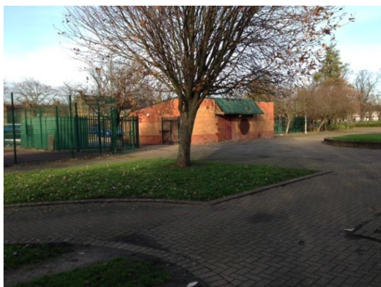
Image 3. Central amenity area and park keepers office.
