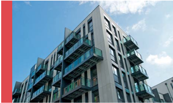
Albermarle Court, Hale Village (photograph: Newlon Housing Trust)
