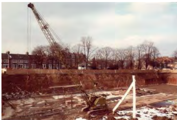
Image 24: Excavation, winter 1984-85 (courtesy of Elaine Norman)
