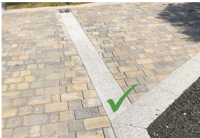
Dish gully replacement - Chesnut Road
