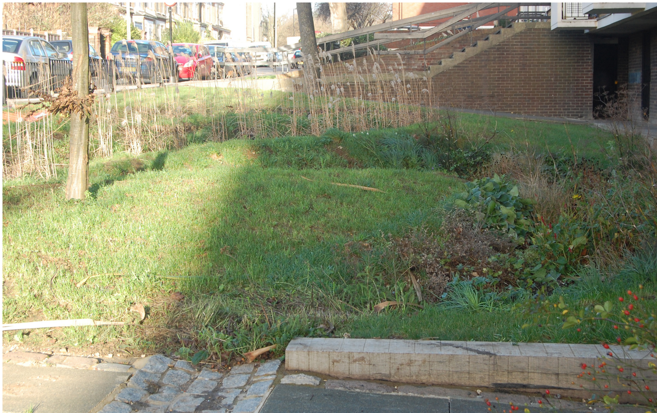
SuDS – Boyton Road
