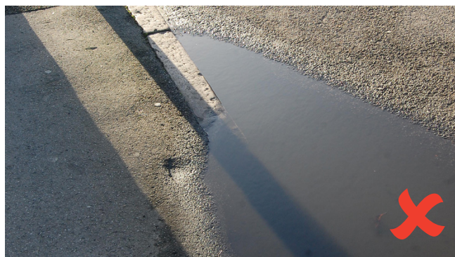
Prevent ponding at crossing points
