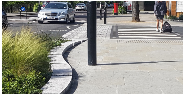
Footway and crossing - Dalgarno Gardens
