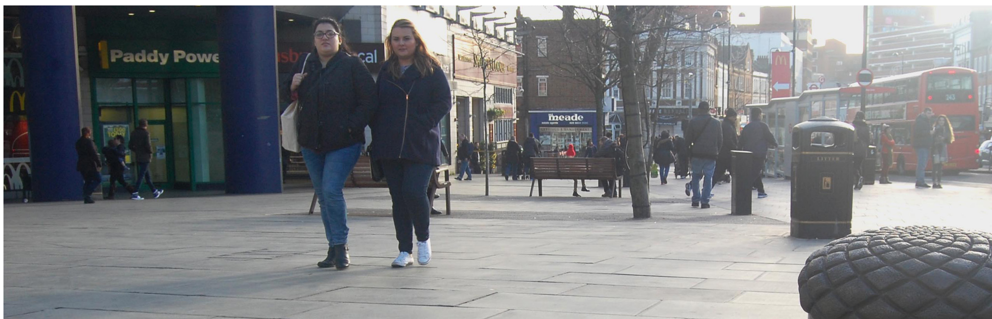
Pedestrian paving and agglomerate - Wood Green Town Centre
