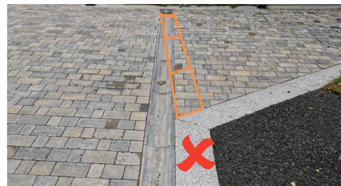
Dish gully replacement - Chesnut Road, Tottenham
