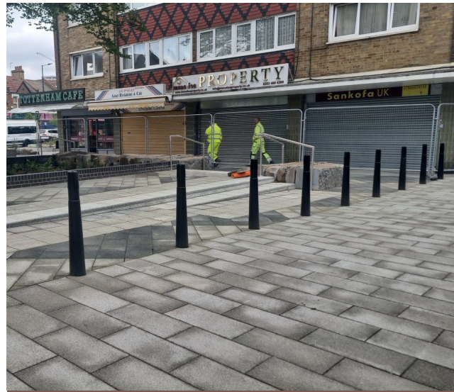
Bollards in Broad Lane
