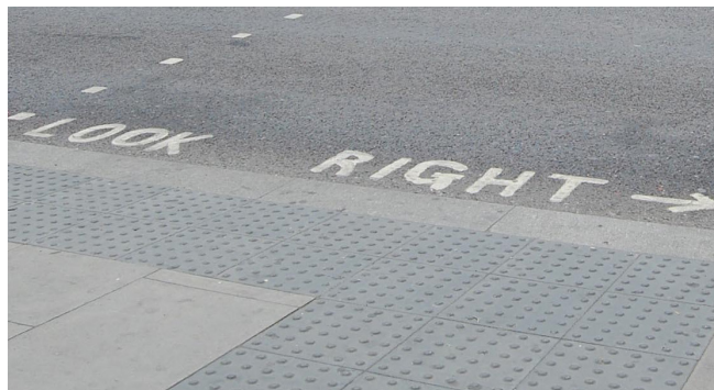
Tactile paving - High Road (A10)
