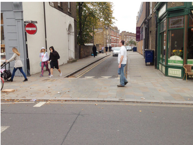
Continuous footways - Old Clapham Town (PCL)
