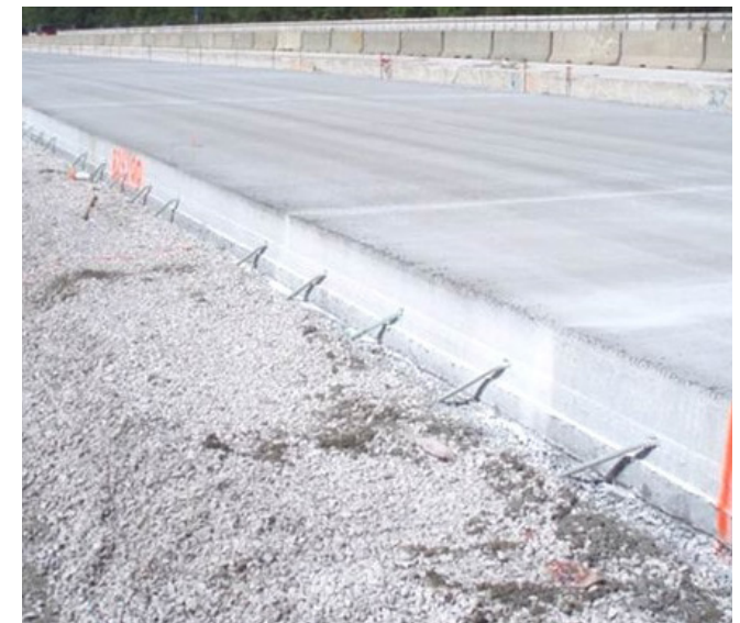
Reinforced concrete under the paving layer
