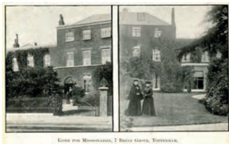
7 Bruce Grove c1907 with low brick walls, brick gate piers and wrought- and cast-iron railings and gates. The view to the right shows the rear of the property.
