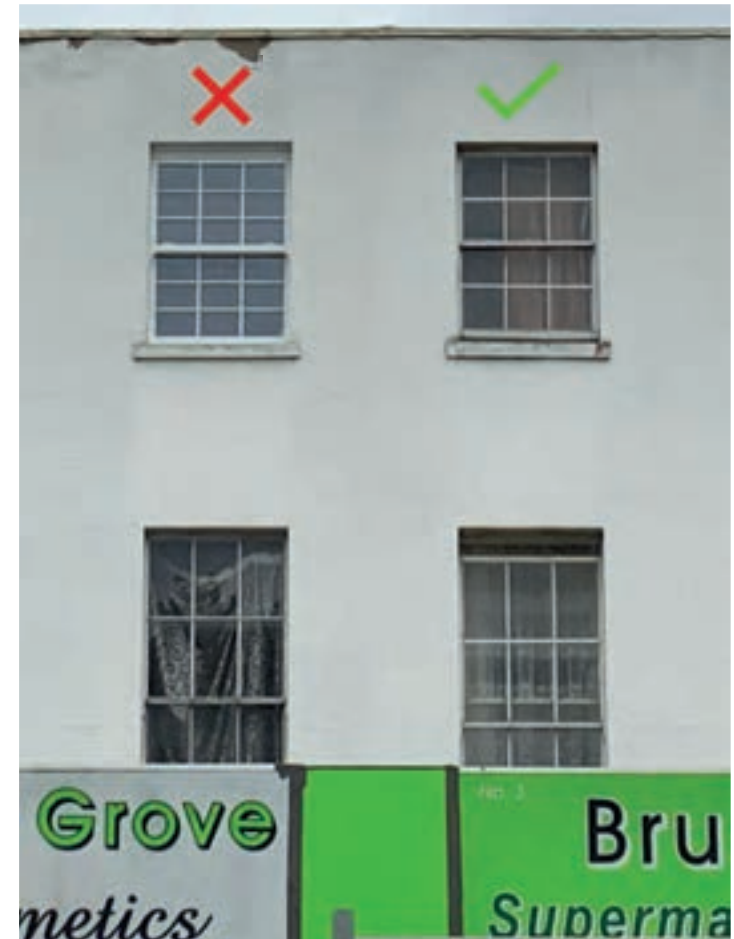
Nos 2 and 3 Bruce Grove; later windows (right) have subverted the original 6-over-6 fenestration pattern (left) with 9-over-9, which is proportionally incorrect and should be replaced with historically correct timber versions to maintain the rhythm of the façades
