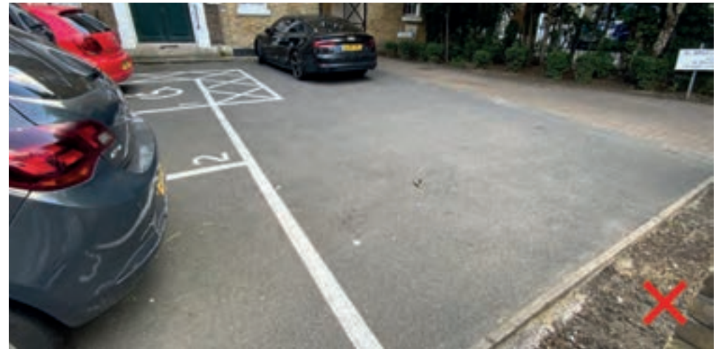
Parking spaces on Bruce Grove delineated by white painted lines add to the 'visual noise' of the forecourts and are at odds with the historic character of the buildings behind
