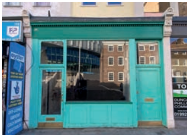
Retained and restored original features (such as these seen in Tottenham) provide clarity to individual components and cohesion to the shopfront design, adding to the character of the shopfront and wider area
