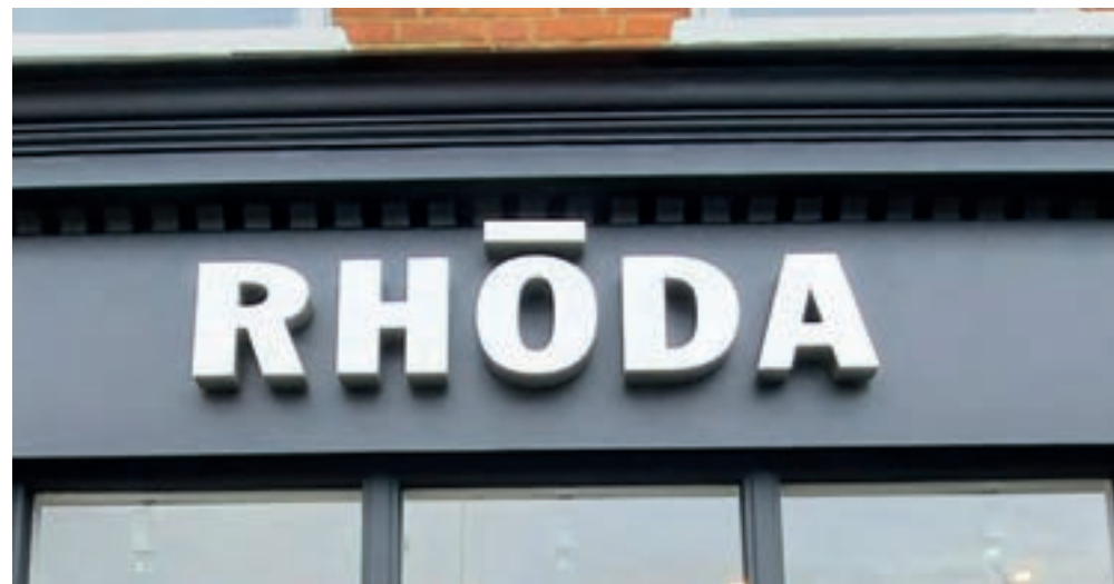
Individual letters applied to the fascia can be appropriate in historic contexts, as shown here in Crouch End
