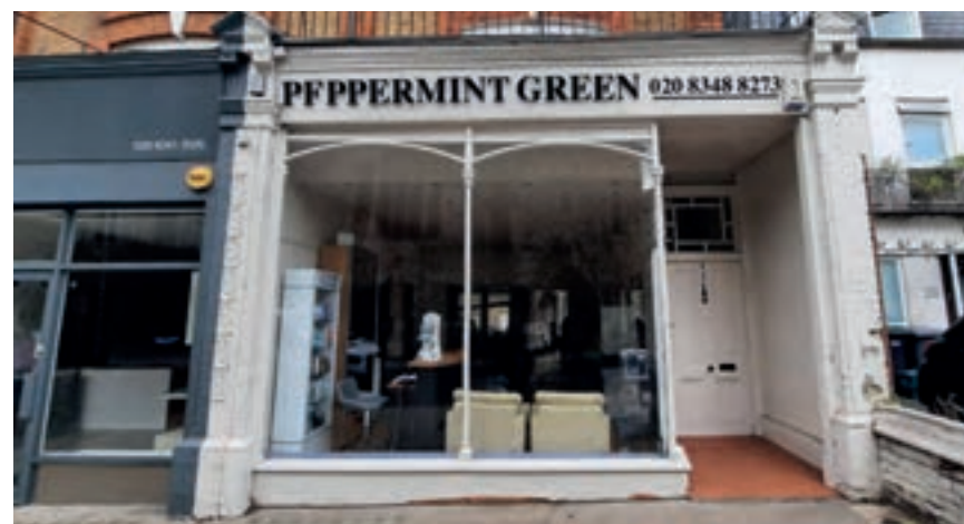
Arched heads and carved capitals and bases to mullions can be used to great effect to embellish shop windows (such as these in Crouch End)
