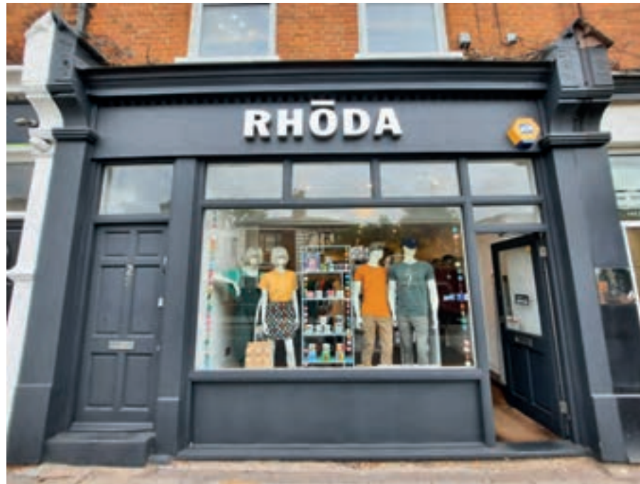
This fascia in Crouch End contains the signage above the shop window and frames the shopfront
