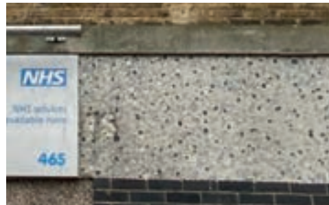
Surviving 1960s mosaic tiling to shopfront, St Mark's Methodist Church, High Road
