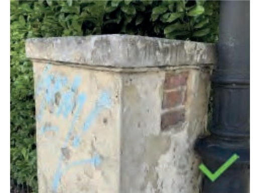
Surviving brick piers with stone capping on Bruce Grove, with metal corner reinforcement on the right
