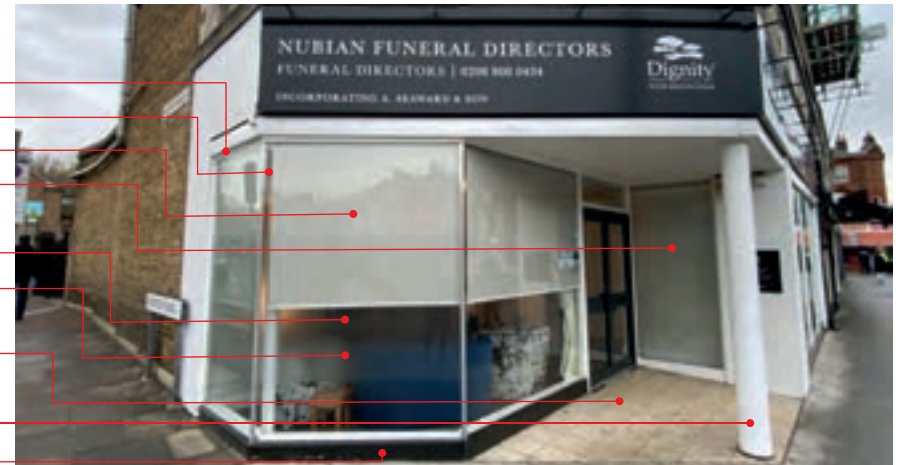
Surviving Art Deco shopfront to St Mark's Methodist Church, High Road; note the flush surround, low stall risers and terrazzo tiles to the entrance lobby floor
