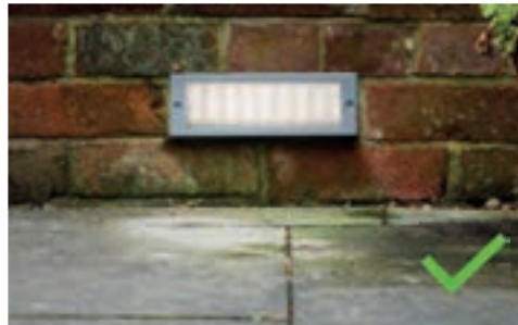
Low-level brick lights can be recessed into walls/piers to illuminate adjacent surfaces whilst being unobtrusive
