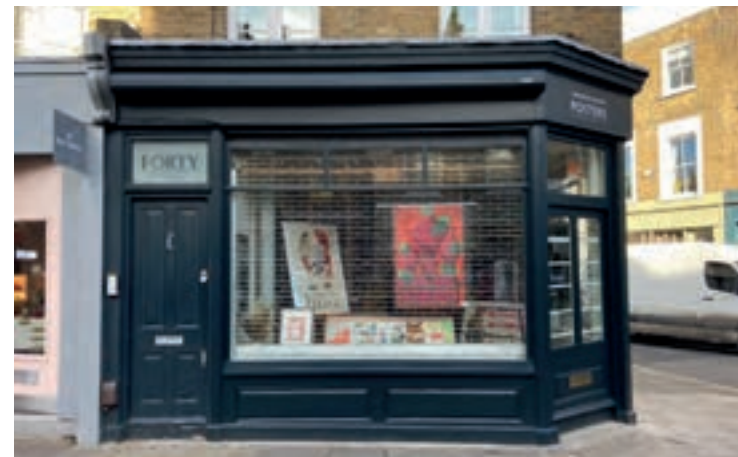
Open grilles placed internally maintain the shopfront free of clutter and allow the shop display to be seen outside of opening hours, as seen here in Crouch End
