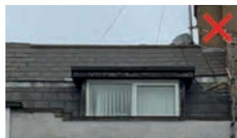
Fascias and bargeboards such as these seen in Tottenham can make dormers appear 'top heavy'
