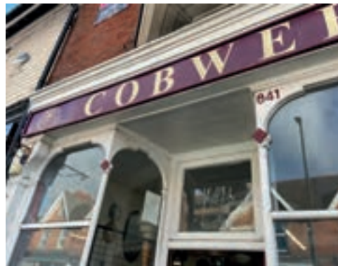
The Edwardians continued with large sheets of glass, with the timber frame featuring slender colonettes forming the mullions coupled with carved spandrels.
