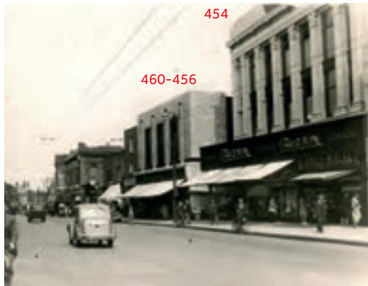
Tottenham High Road looking north from St Loy's Road, 1947
