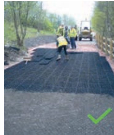
Products such as 'Grasscrete' or similar maximize amenity whilst providing robust surfacing that is low maintenance and suitable for vehicles
