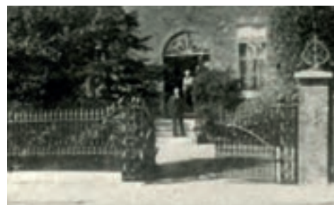
No. 7 Bruce Grove c1907 showing typical boundary treatment with brick piers and iron gates and low brick walls with iron fencing to the top, with planting set behind
