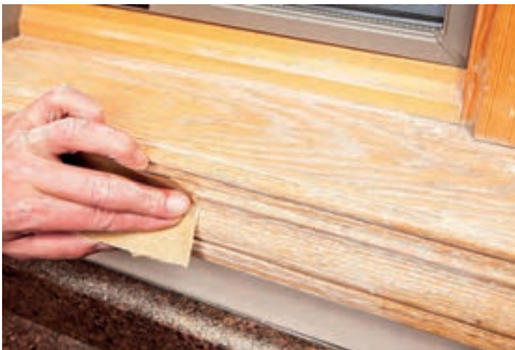
Timber surfaces should be lightly sanded prior to painting.
