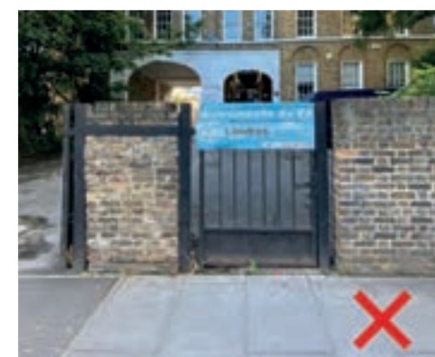
Higher boundary walls on Bruce Grove obscure views of building façades and present an unattractive aspect to the paving
