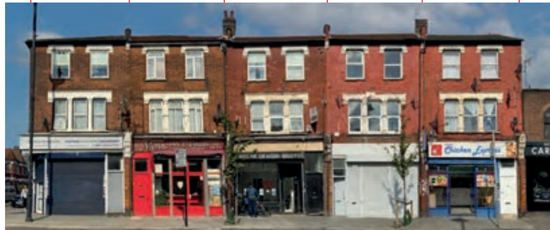
SURVIVING EARLY TIMBER SHOPFRONT EDWARDIAN (BUILT 1905)
