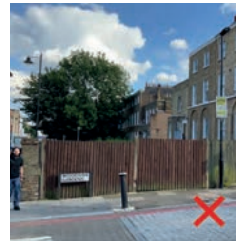
Modern timber and concrete fences on Bruce Grove are at odds with the historic character of the houses
