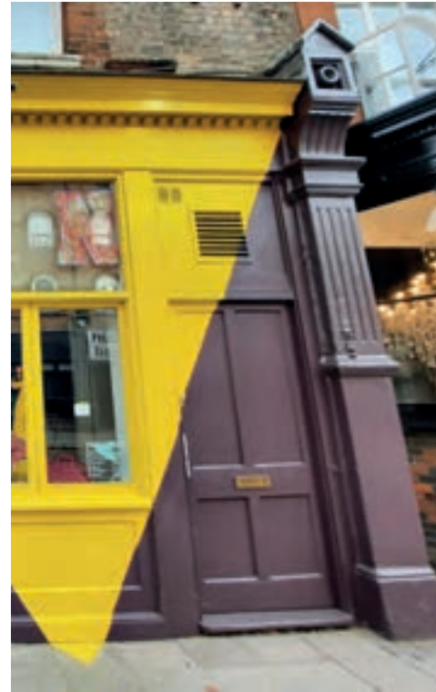
Console brackets, cornice, fascia, pilasters, plinth and stall riser working together in a complete composition (Crouch End)
