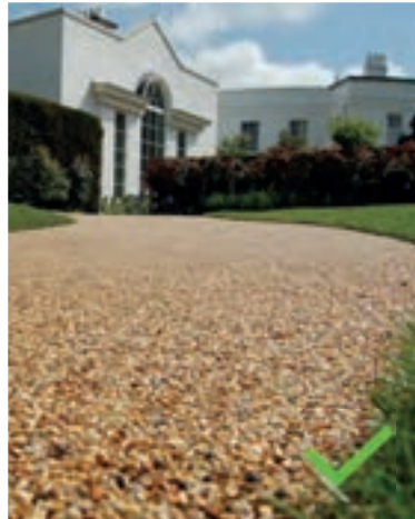
Resin-bound gravel in conjunction with stone cobbles provides a sympathetic modern surfacing that complements the character of the historic context
