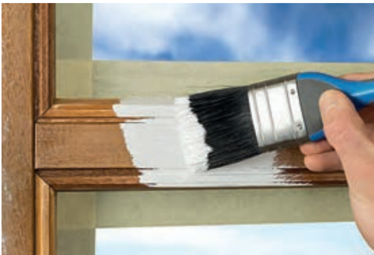
Apply paint evenly and according to manufacturer's instructions.
