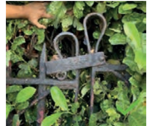
Original carriage gates at 16 Bruce Grove
