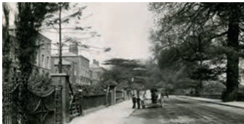
Bruce Grove, c1900, looking north west, with the houses at Nos 5 to 16 to the left and elm trees to the right. Note the low brick walls, brick gate piers, wrought and cast-iron railings and gates, and timber gates.
