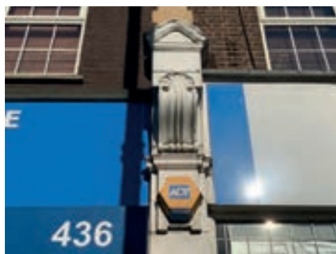
Alarm boxes and sounders should not obscure architectural features, as seen here in Tottenham
