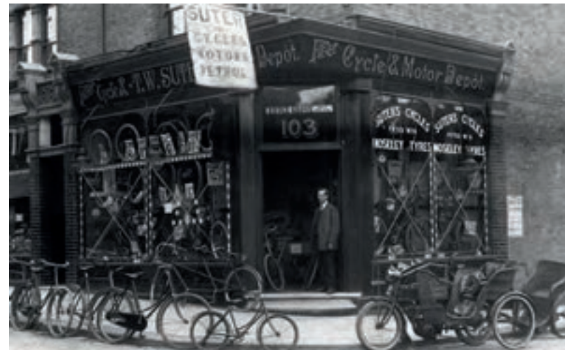
Edwardian shopfront to No 103 Bruce Grove, c1905
