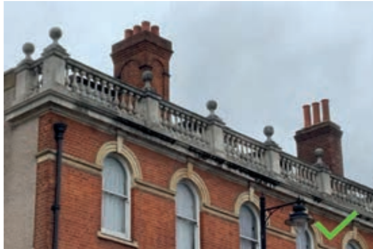
Chimney stacks like these in Tottenham are important features of the roofscape and can be key indicators of the date of a building and of the internal planning. These should never be removed or altered without consent
