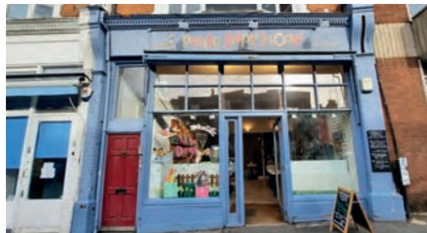
Smaller pane windows with mullions (vertical framing elements) and transoms (horizontal framing elements) as shown here in Crouch End add visual interest, improve security and are easier to replace if broken
