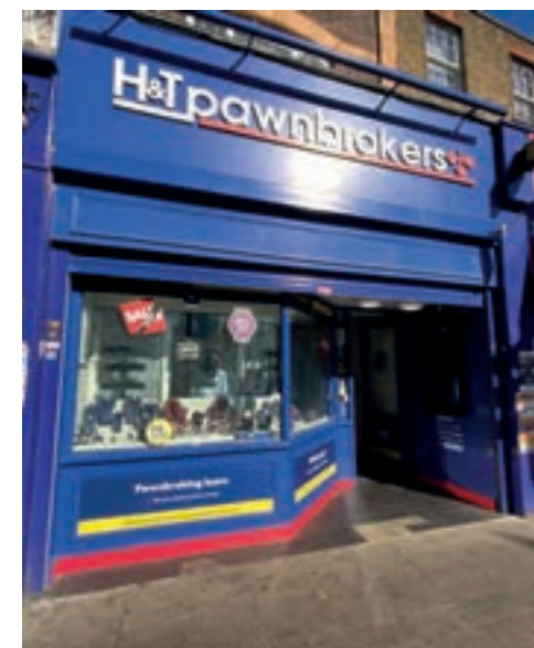
The use of a recessed doorway and ramp can provide level access and enable doors to be opened in both directions, as shown here in Tottenham
