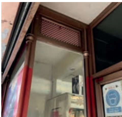
Ventilation grille contained within the transom light at the top of a shop window in Tottenham
