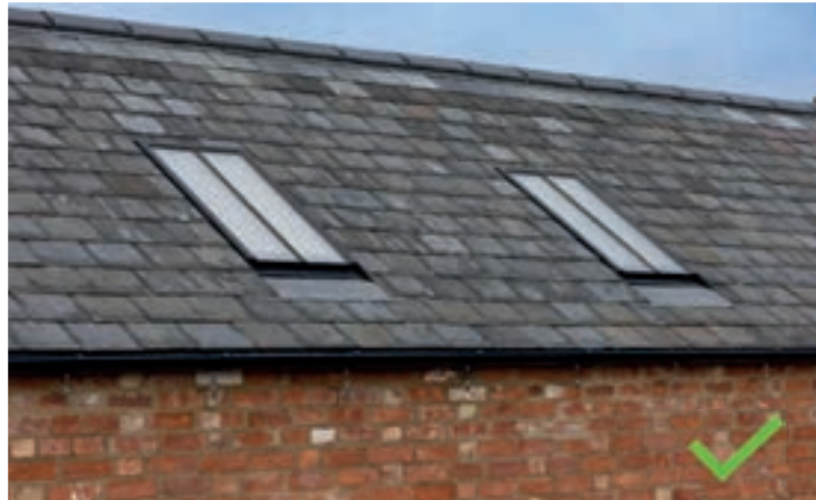
Rooflights should be of the 'conservation' type, flush with the surrounding roof surface and with larger panes of glass broken down into smaller sections with glazing bars.
