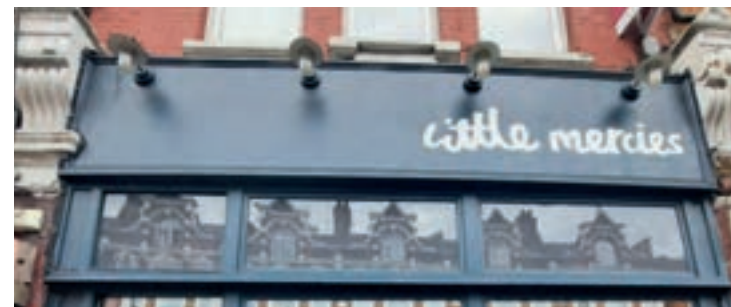
Services should have concealed cable and pipe runs, as seen here in Crouch End
