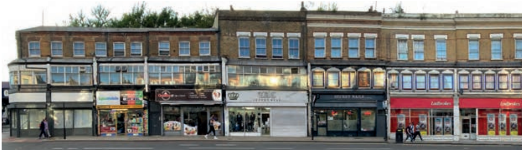
MID-C19 WITH LATE-C19 SHOPFRONTS/WINTER GARDENS
