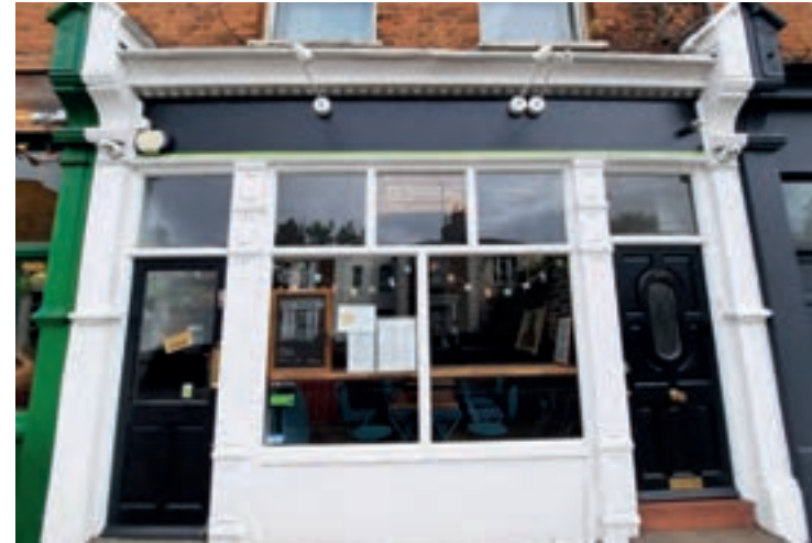
Smaller-pane glazing like that shown here in Crouch End is more difficult to break, less of a target to vandals and easier to replace if broken
