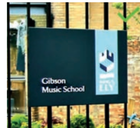
Signage may be fixed to railings but should be 50 x 50 cm maximum and of a sympathetic design that does not detract from the historic context.
