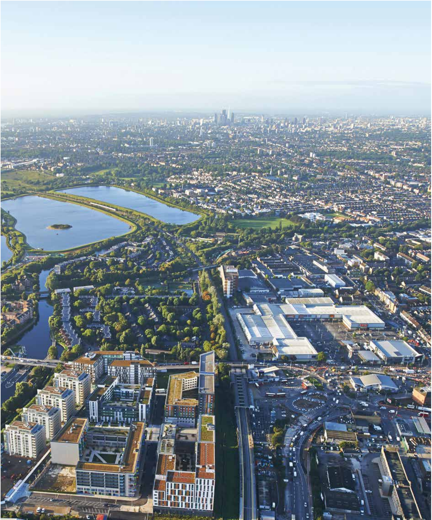
Aerial view of Tottenham Hale looking south
