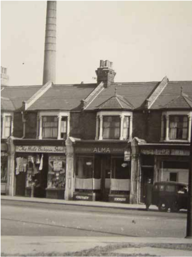
The Hale and factory chimney, 1955
