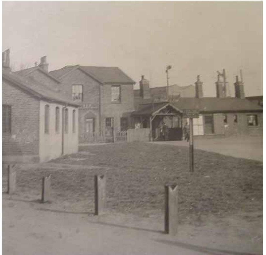
The Hale and factory chimney, 1955
