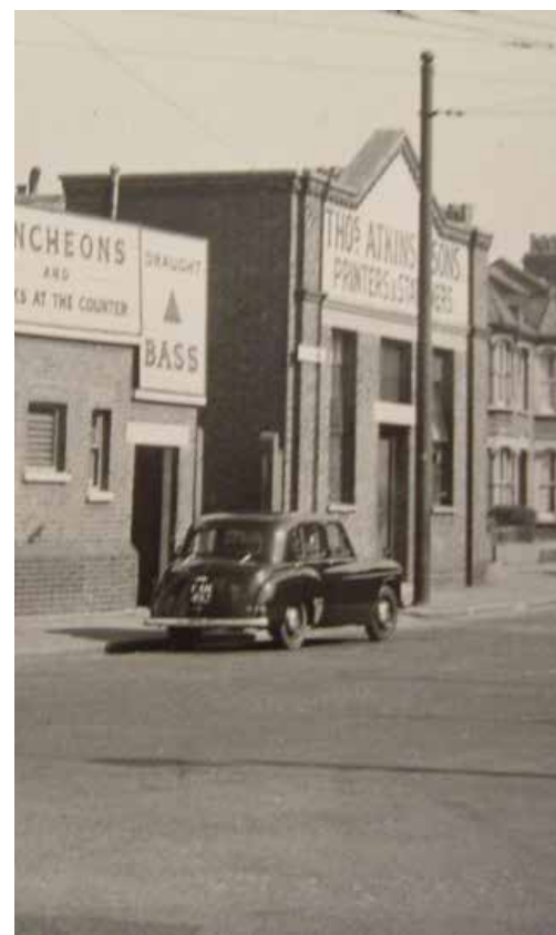
Station Road, looking west, 1955
