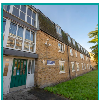
Bedale House 23 Boyton Road, N8 7AZ
