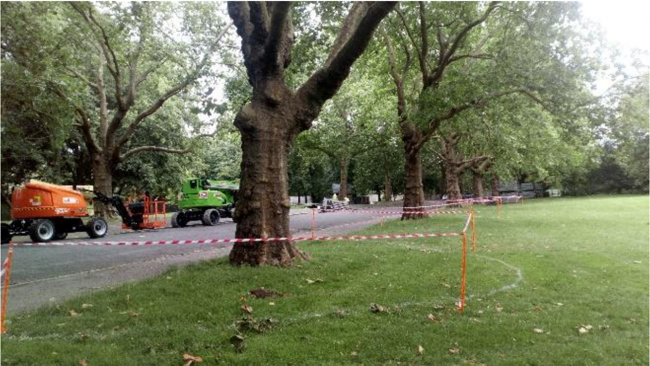
Figure 1: London plane avenue with tree protection areas marked by barrier tape for duration of pre-event build period and post-event break period
