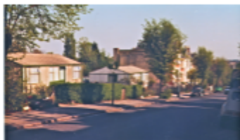
Granville Road prefabs, April 1947 (Courtesy Alexander Smith, local resident)
