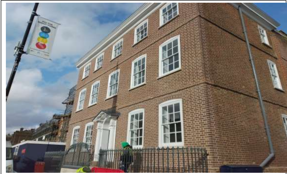
Dial House, 790 High Road, with restoration almost complete (work continuing on Northumberland Terrace in background)
