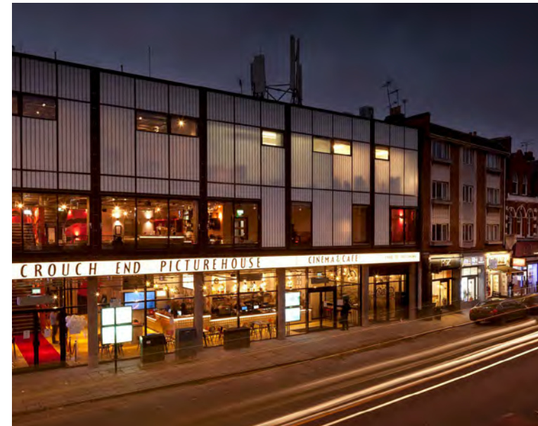
Crouch End Picture House, Panter Hudspith Architects Haringey Design Award 2016 - Best Green Design
