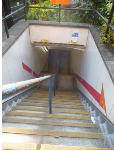
Photo 12: Southwood Lane Tunnel (entrance)
