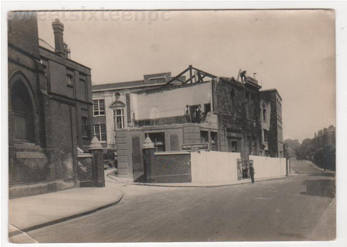
Photo 1: former British School (being demolished)
