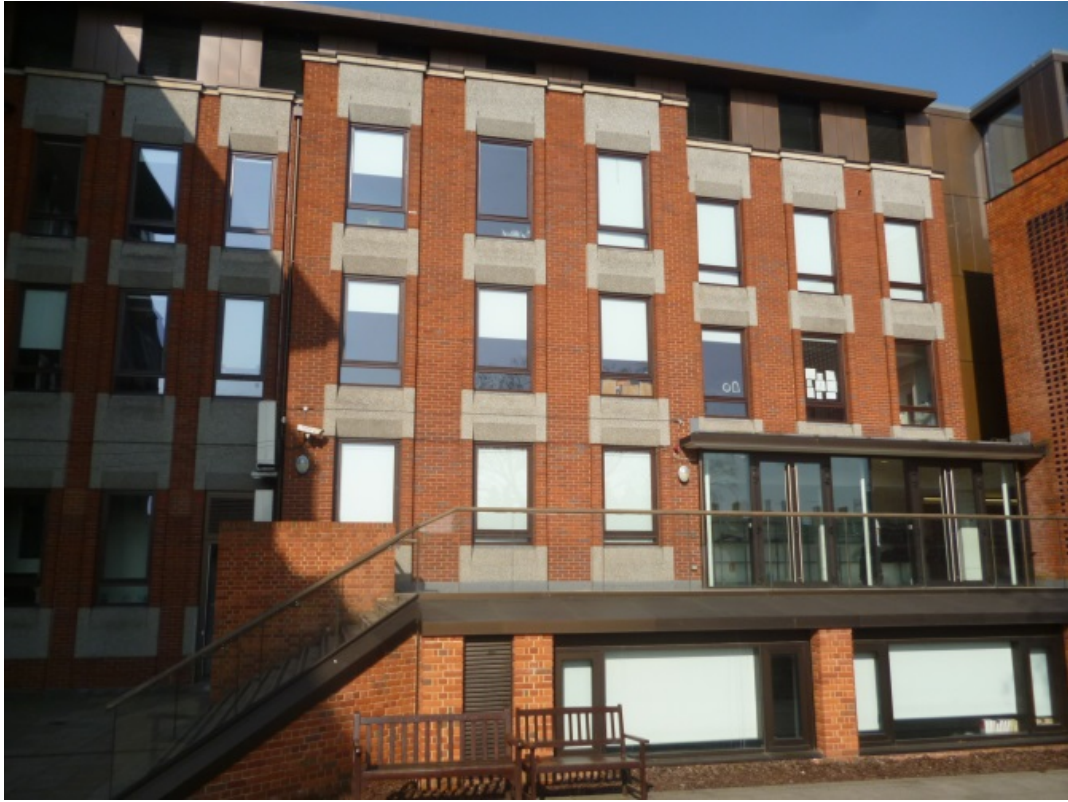
Photo 6: Garner Building (rear)
