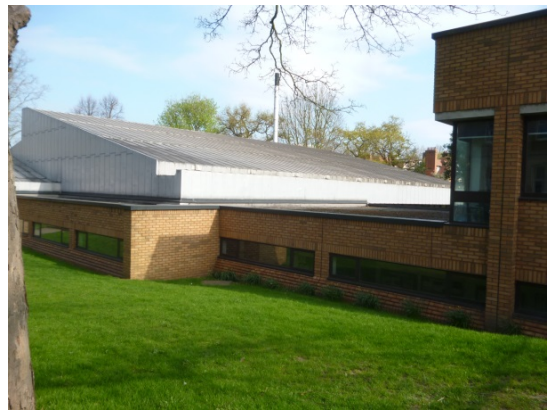
Photo 21: Swimming Pool (Mallinson Sports Centre)
