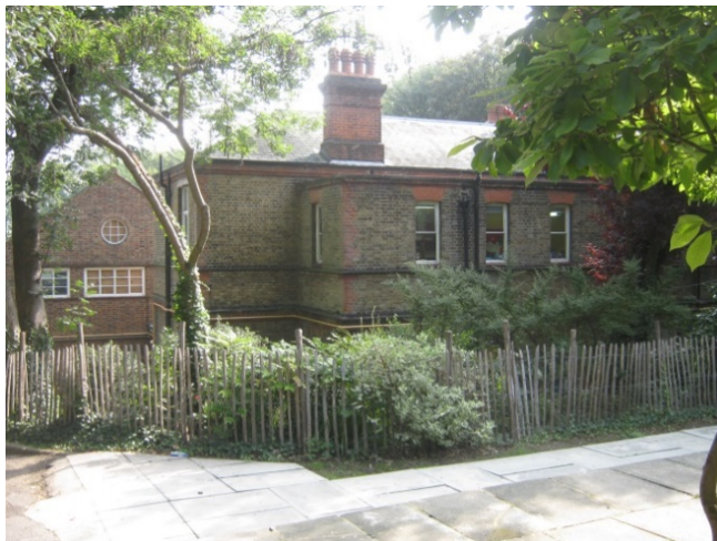
Photo 9: Classroom Block (Dyne House Site)
