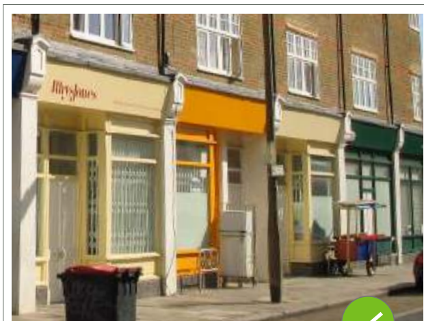
Internal shutters which don't obscure architectural features
