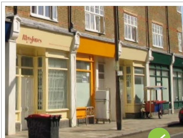
Internal shutters which don't obscure architectural features
