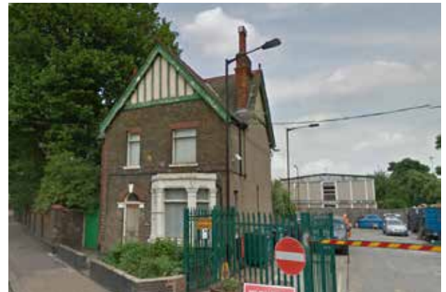
Victorian house on the depot site opposite Carew Road
