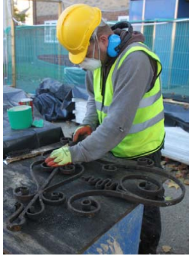
Restoring wrought iron sign bracket.
