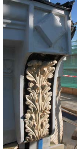
Restored corbel above shopfront.
